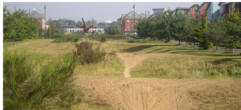
SuDS infiltration basins have been integrated with highways at Ravenswood in Ipswich. The scheme is estimated to have saved over £600,000 in the long term (Ipswich Borough Council, 2011)
