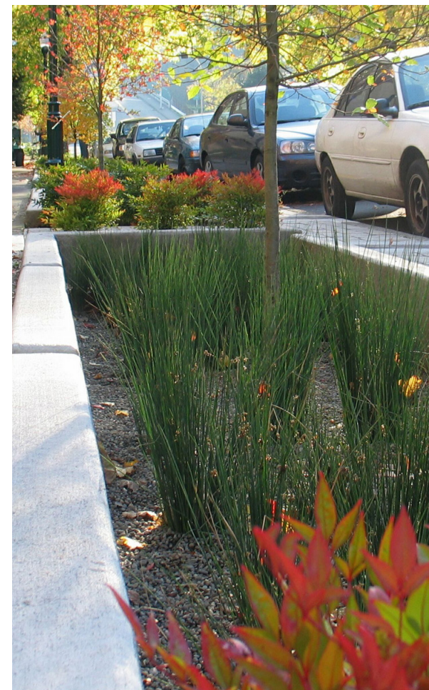
Bio-retention planters, Portland, Oregon, USA
