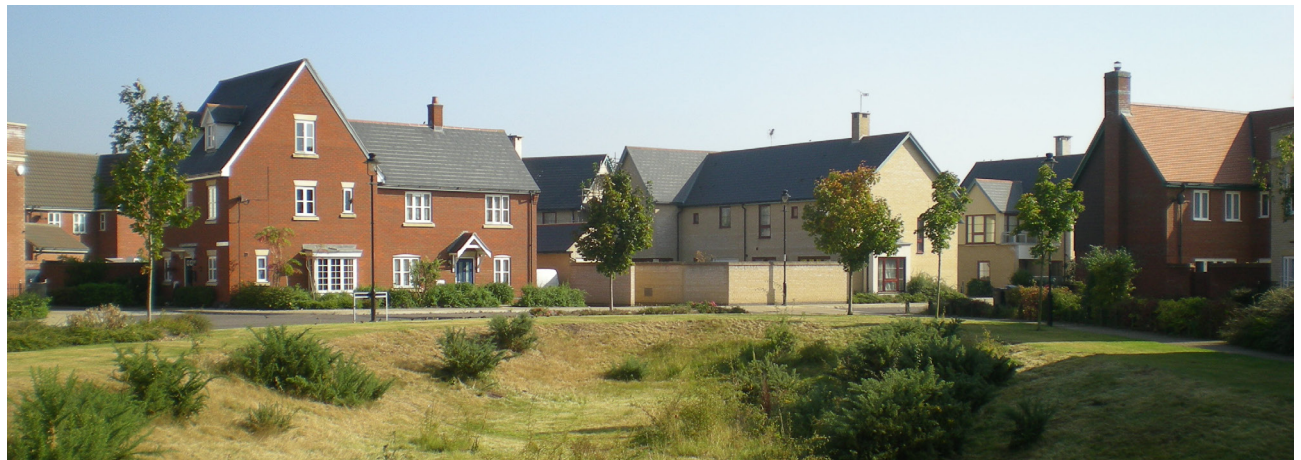
Infiltration basin at Ravenswood, Ipswich, Suffolk.
